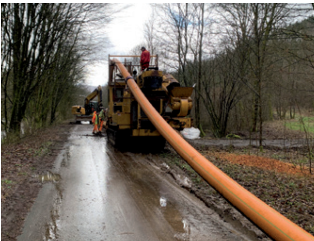
Installation of the pipeline by trench cutting
