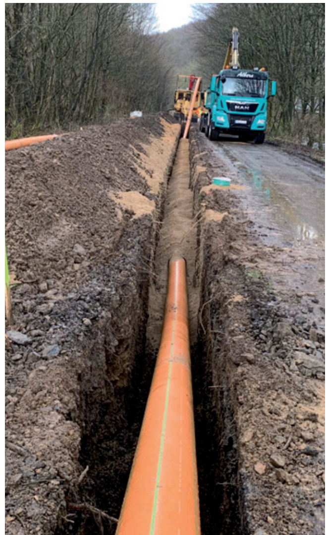
Pipe insertion into the pre-cut trench
