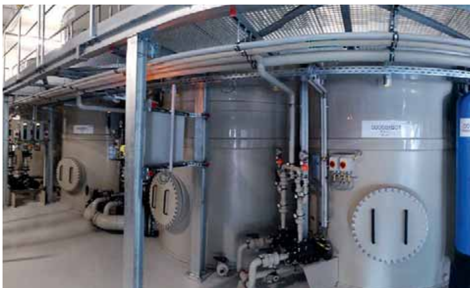
Intelligent pipe systems made of PE, PP, PVDF for process water and wastewater treatment
