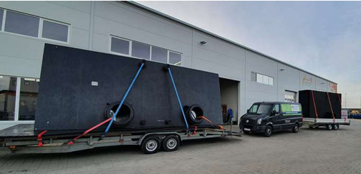
From left to right: transporting the individual components of the 100 m 3 plastic tank to the incampus energy centre; a telehandler placing the front wall in the incampus energy centre; erection, assembly and welding of the individual components on site
