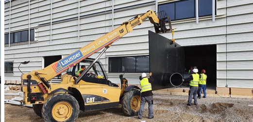
From left to right: transporting the individual components of the 100 m 3 plastic tank to the incampus energy centre; a telehandler placing the front wall in the incampus energy centre; erection, assembly and welding of the individual components on site
