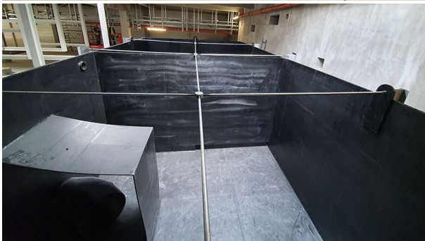
Top: ready-assembled 100 m 3 cooling water tank made of cross-ribbed SIMONA® PE 100 black Twin-Wall Sheets; bottom left: plastic tank with a bolted steel frame made of galvanised steel IPE sections; bottom right: cross-ribbed SIMONA® PE 100 black Twin-Wall Sheet
